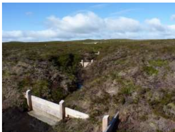
Slowing runoff to restore peatland
